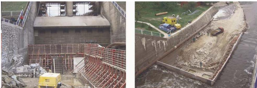
Figure 10. Upstream and downstream view of stilling basin of the Znojmo dam; a part of the basin is under the cofferdam and the preparation of fabrication of baffle blocks is in progress
